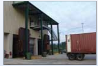
This transfer station, located in Salem, VA, features two BlokPak 3000 compactors for non-stop processing as well as added redundancy. They are fed from a tipping floor.
